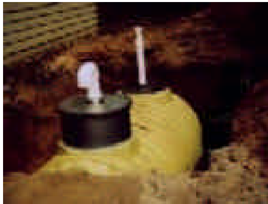
Figure 3: Exterior picture of the Life Pod unit placed into the ground.
